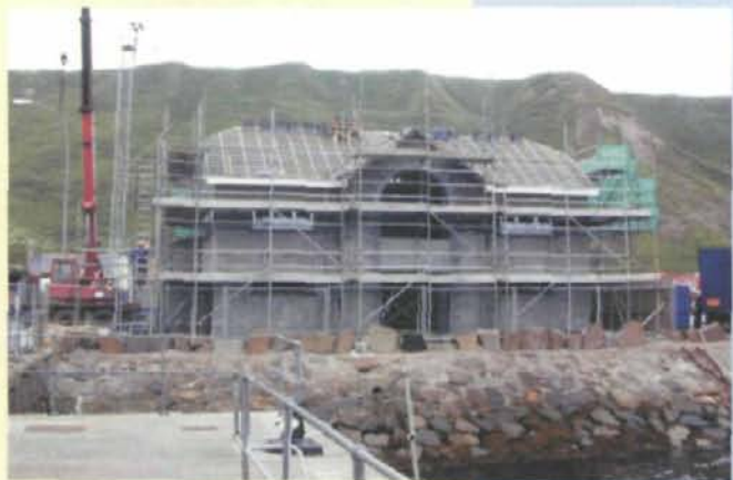
Below: Construction of the new facilities at Thurso.
