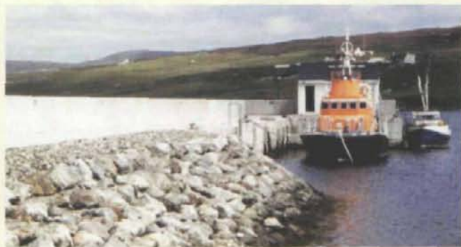
Below: The breakwater at Aith giving shelter to the station's Arun class.
