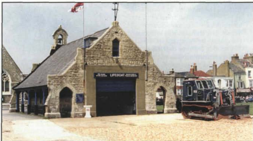
Walmer's boathouse was designed by the RNLI's first Honorary Architect, Charles Cooke. Appointed in 1858 Cooke was influenced by a building he had designed for Colombo (then Ceylon) with overhanging eaves to give protection from the tropical sun.
