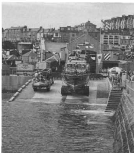
The new boathouse and slip at St Ives, Cornwall
