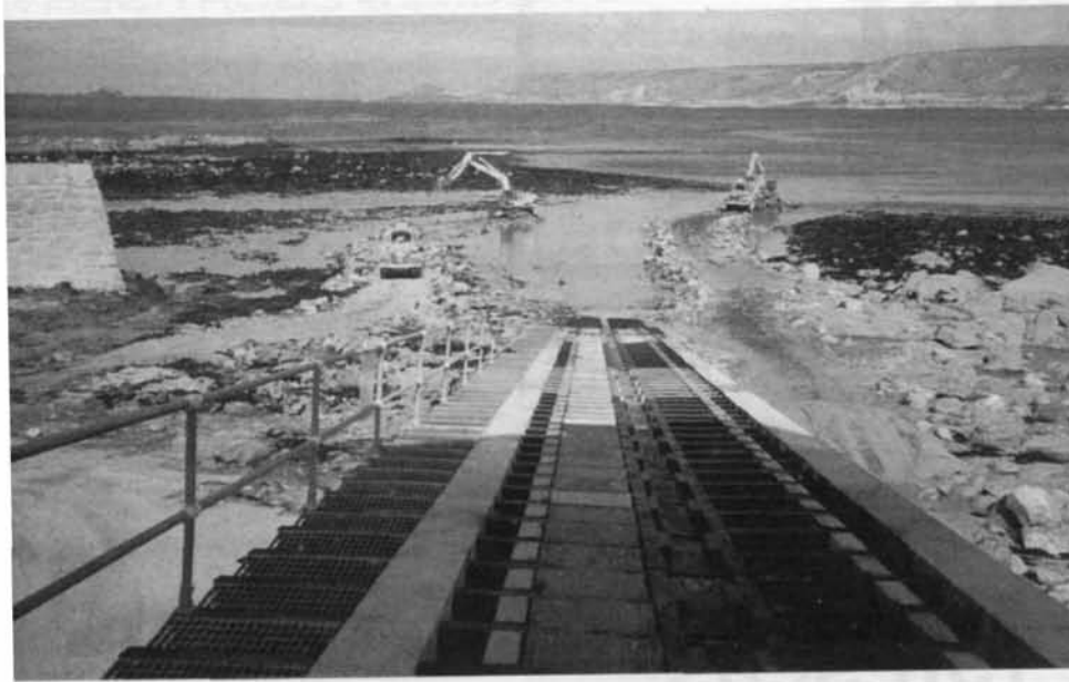
Major shoreworks, such as this dredging to give Sennen Cove's new Mersey less launching restriction is the kind of expense which normally has to be met from general funds. Legacies to aid this type of work are very valuable. Photo Peter Puddiphatt
