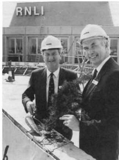
Lt Cdr Brian Miles, director of the RNLI, (left) and the managing director of Laing's, Trevor Berry, lay the highest section of concrete to mark the topping-out of the RNLI's new headquarters building. (Photo Southern Newspapers)
