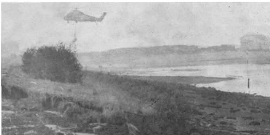
Wells: Roadway to lifeboat house (r.) was washed away in two places. RAF Wessex helicopter ferries sandbags to fill breaks. photograph by courtesy of RNLI Enthusiasts Society, Cromer and District Research Group
