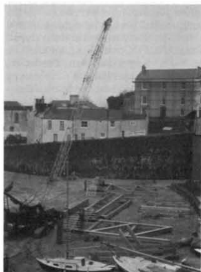
Galvanised steel section columns and bracing members were bolted together on the beach and then (right) lifted into place by crane at low water.
