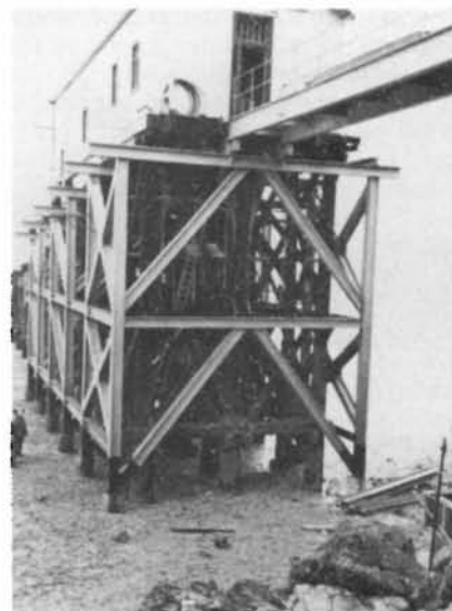
Six 600mm diameter tubular steel piles were driven on each side to support the new galvanised steel substructure which was built up before the decayed timber was cut away.
