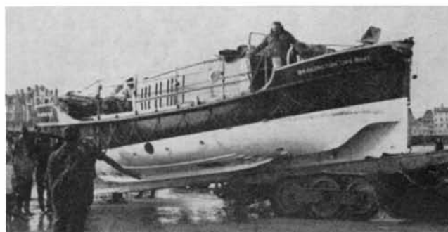
5: . . . channel track of little turntable (left) on which she can be swung round to convenient position for mounting on carriage. Tractor moves round carriage . . .
