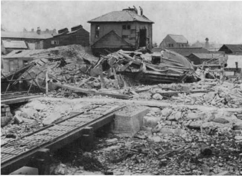
A direct hit on the lifeboathouse and lifeboat at Tynemouth on April 9, 1941. The heavy bomb, with a slightly delayed fuse, penetrated and exploded under the concrete floor. by courtesy of J. C. H. Cleet
