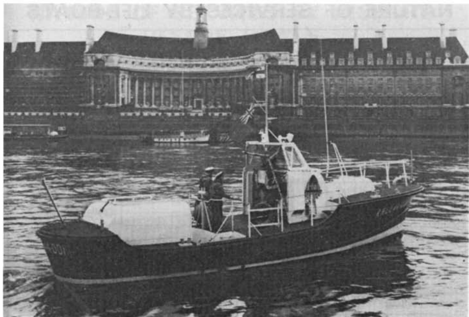
The new 44-foot steel life-boat in the Thames at London
