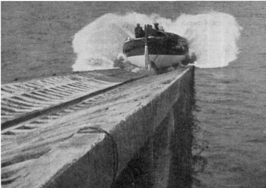
LAUNCHING BY SLIPWAY. The Motor Life-boat Edward, Prince of Wales , at the Mumbles.
