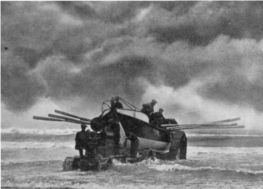
LAUNCHING BY TRACTOR. The Aberdeen Pulling and Sailing Life-boat
